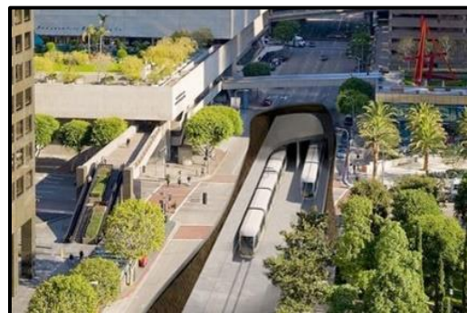
Flower Street Box Tunnel
